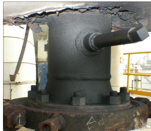
**THURMALOX 837/225HD** — A self curing hybrid inorganic zinc rich primer with a maximum heat resistance of 1200°F (649°C). Endcor 837 topcoated with Thurmalox 225HD is ideal for use on new construction insulated carbon steel surfaces.
