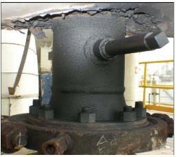
**THURMALOX 837/225HD** — A self curing hybrid inorganic zinc rich primer with a maximum heat resistance of 1200°F (649°C). Endcor 837 topcoated with Thurmalox 225HD is ideal for use on new construction insulated carbon steel surfaces.
