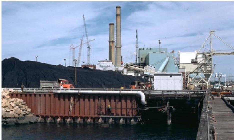
Seaward corner of the coal-unloading pier is shown completely primed with Epodur®2755 primer, a moisture-tolerant corrosion inhibitive primer that cures rapidly and allows topcoating prior to the rise of the incoming tide
